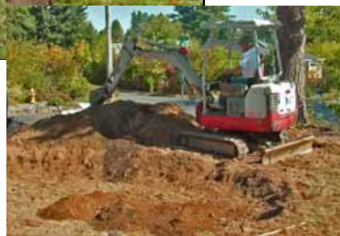
Using a mini-excavator makes the work easier for larger rain gardens.
