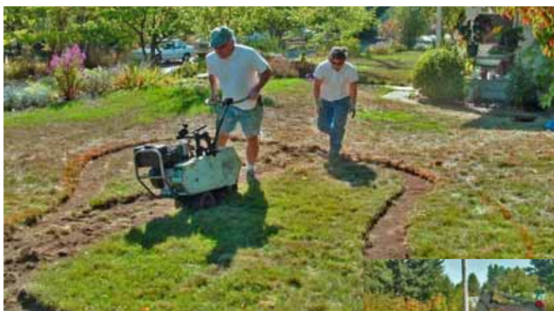
Removing sod with a sod cutter before building the rain garden.
