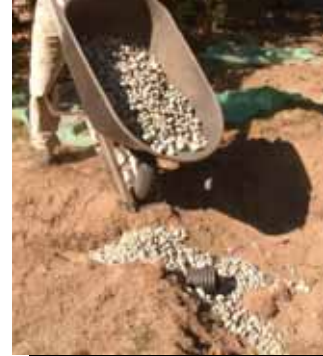
Placing washed rock around inlet
