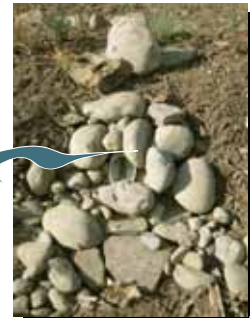
Rock lined inlet. Rock should be free of sediment, so order "washed."
