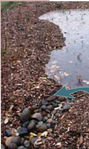
Rock lined overflow
